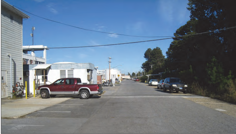
Figure 3-8. Portable Building Behind Hangar 111, Facing East
