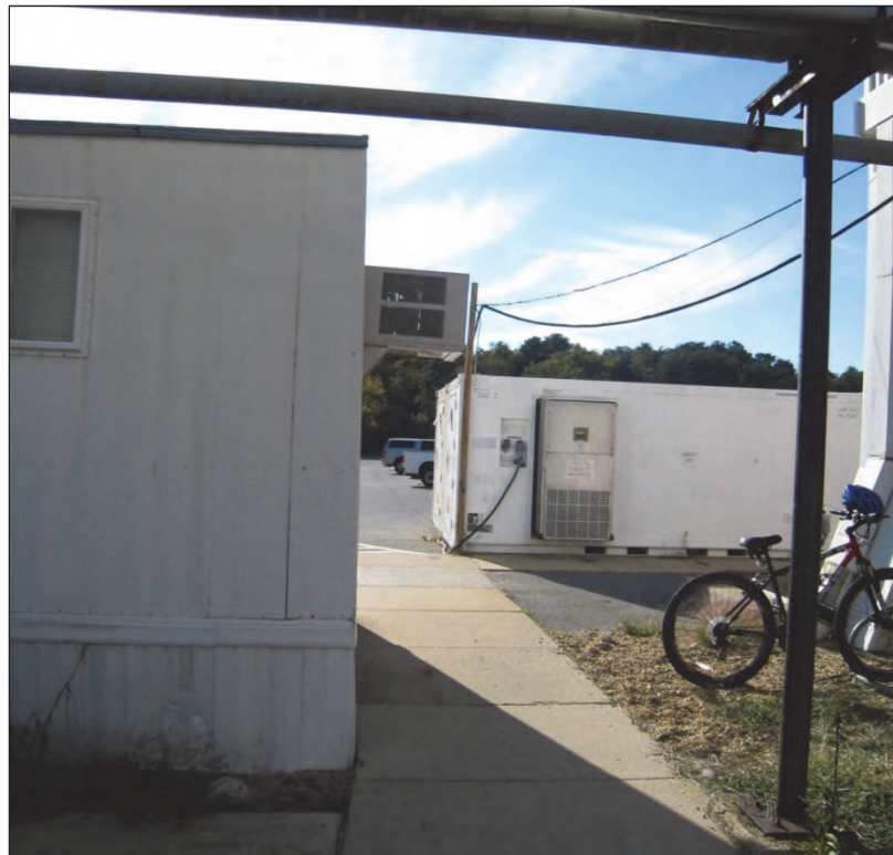
Figure 3-7. Portable Buildings Behind Hangar 111, Facing West
