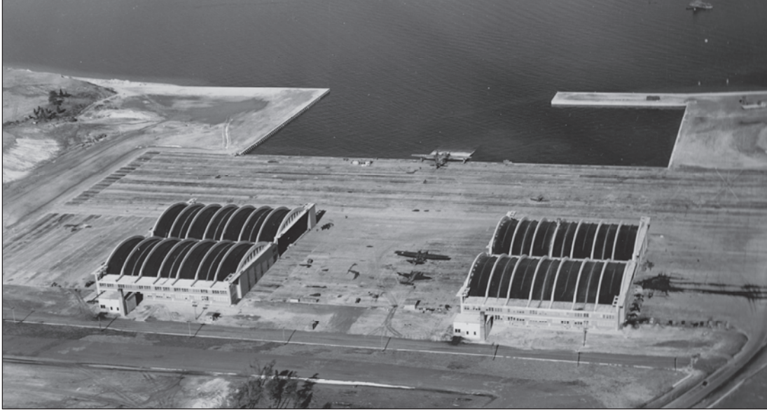
Figure 3-5. Detail of 1944 Photograph of Hangars 111 (left) and 110 (right) and Their Heating Plants 111A and 110A, Facing North
